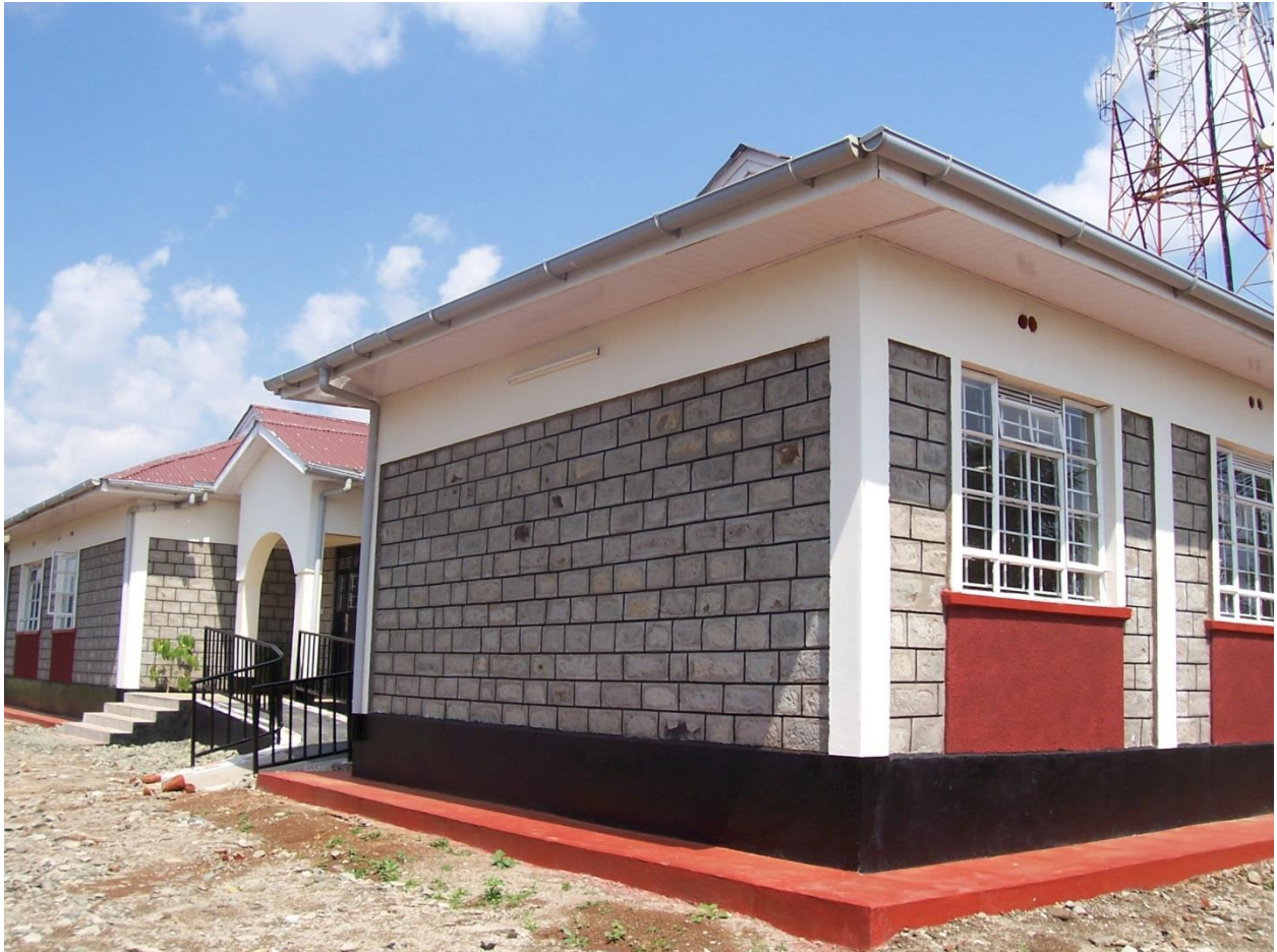
Front view and entrance of the SCL Complex. This is the headquarters of the Integrated Development Africa Programme (IDAP). For our disabled brothers and sisters who may not be able to use the staircase, we have a very friendly access route into the building.
